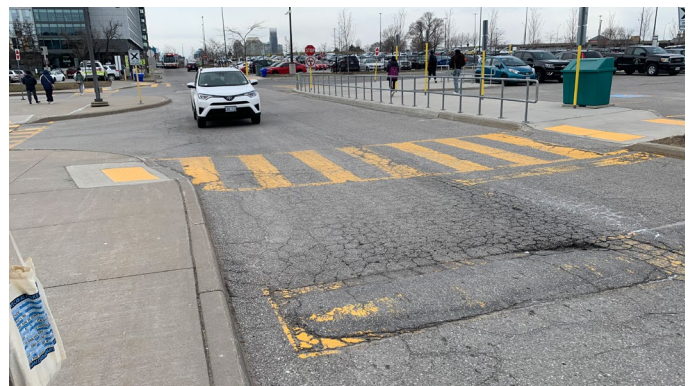
Pedestrian and cycling infrastructure not prioritized on campus
